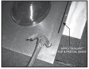
Figure 10.21 Slide Flashing Down, Secure & Apply Sealant
